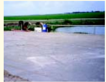
Wash pad with collection pond
