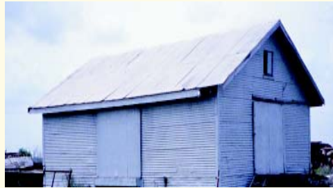
Pesticide storage shed
