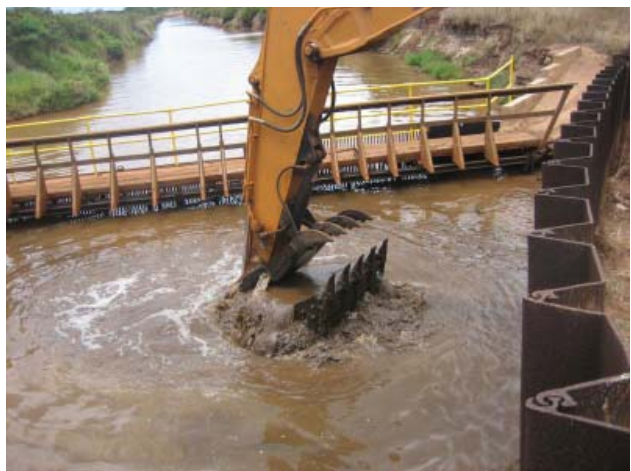
Removal of silt at Kawaiele Pump Station wet well.
