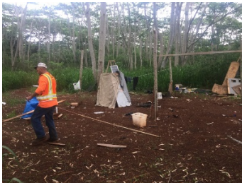
Removal of Encampment & Trash
