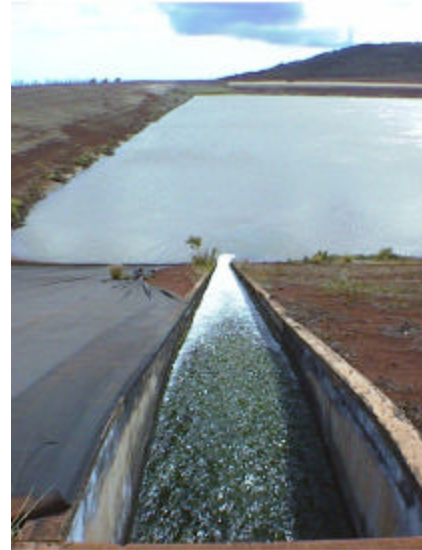
Inlet from the transmission pipeline.
