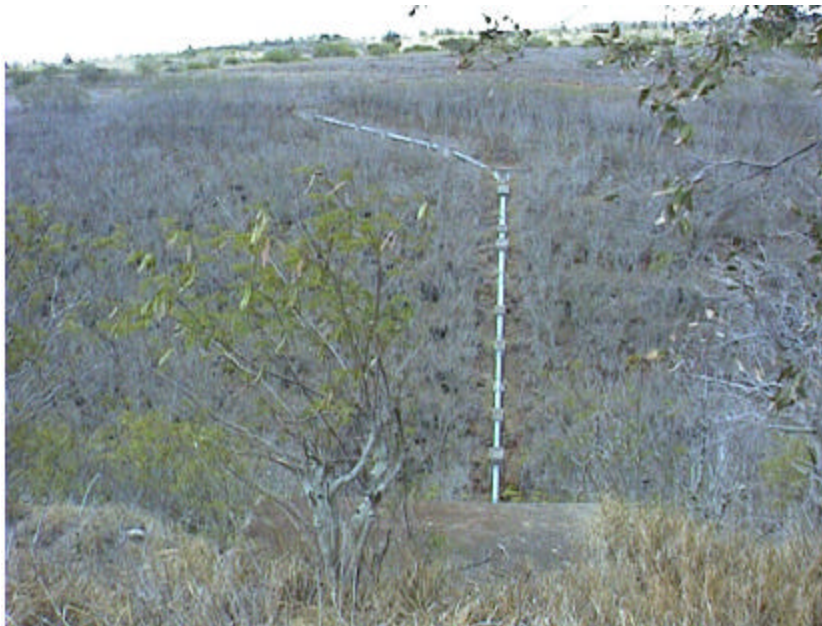
Transmission pipeline heading toward the Kualapuu reservoir.
