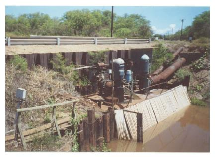
The Nohili pumping station at the Pacific Missile Range Facility (PMRF) on Kauai keeps the Mana plain water table low. During major rain storms, the station helps prevent flooding at the PMRF and in the nearby town of Kekaha.
