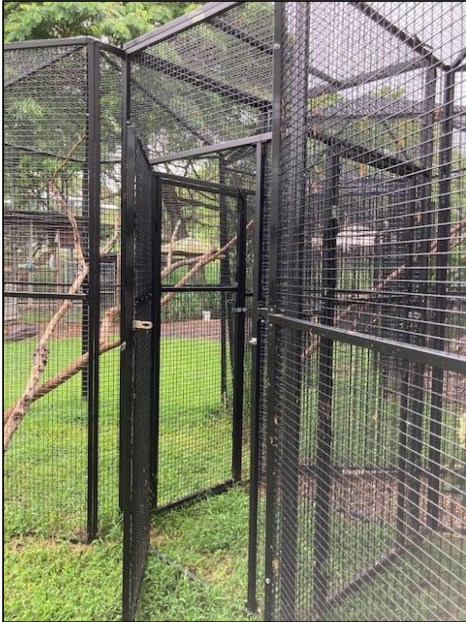
Photograph 11: Depicts the double entry way to enter the new containment structure for the Lemurs.
