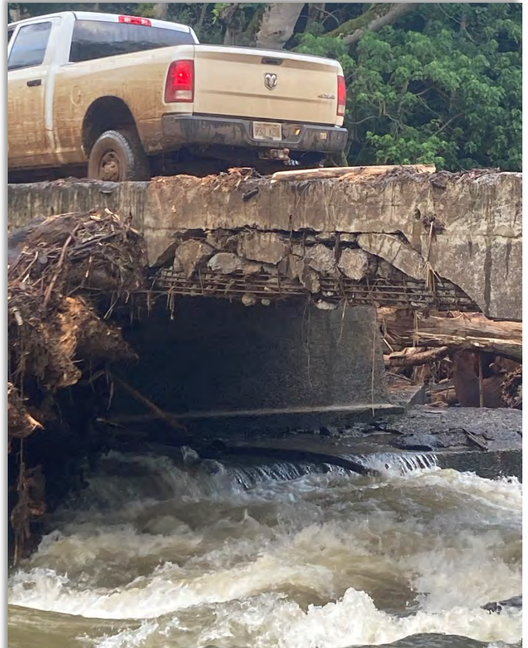
Image 1: Damage to Christian Crossing Bridge from flooding.
