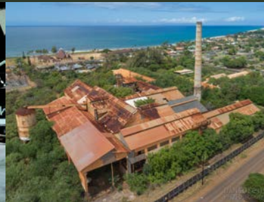
Insufficient Processing Plant
